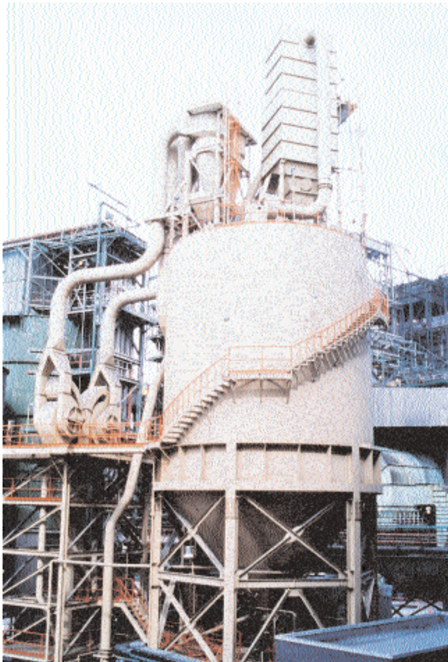
Once classified, the in-spec fly ash is conveyed to a 1,300-ton storage silo for unloading to trucks for bulk shipment.
